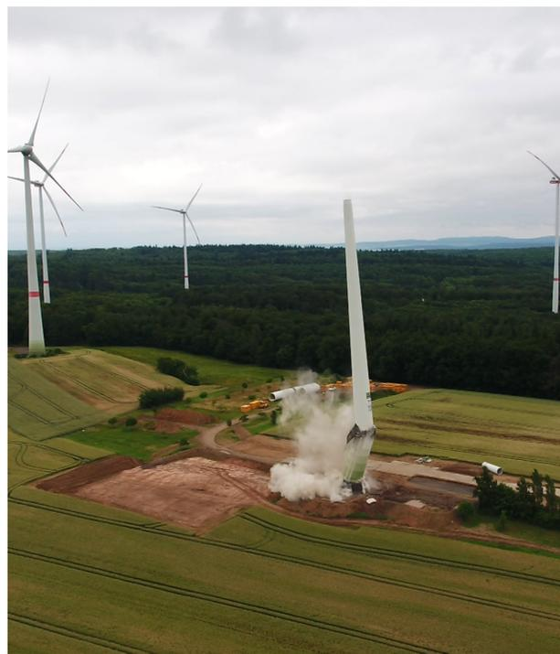
Fig. 1: Execution of a tower demolition using the folding blast method. Using a second explosive charge at 1/3 of the total height, the upper part of the tower collapsed in the opposite direction to the lower part. This method is more space-saving than a conventional tower collapse blasting. © Reisch Sprengtechnik GmbH
