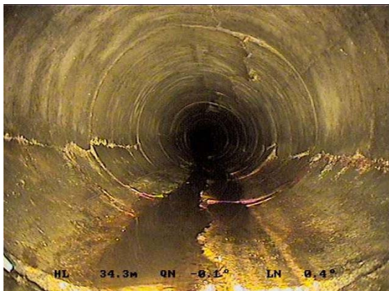
Fig. 10. Video print of the airport sewer DN 700
