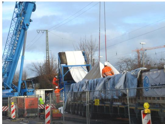
Figure 22. Installation of the CIPP lining
