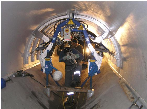
Figure 15. Erection device to press the 4 m long polyethylene sheets against the culvert
