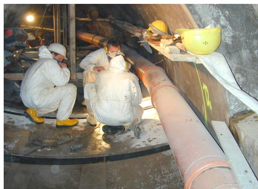
Figure 20. Assembly of the liner elements, bonding
