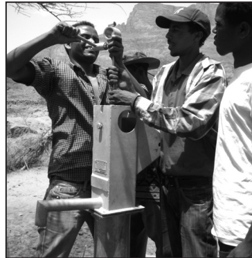
Fig. 8 | Installation of the hand-pump (type: AFRIDEV) (Foto: KLOPPER 2009)
