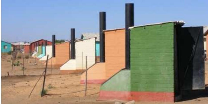
Abbildung 37: Otji-Toiletten in Otjiwarongo (ClayHouseProject, Clay House Project)
