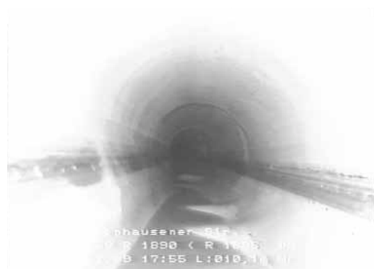
Figure 15. Transverse folds in re-deformed lining
