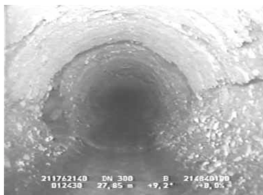
Figure 11. Concrete corrosion
