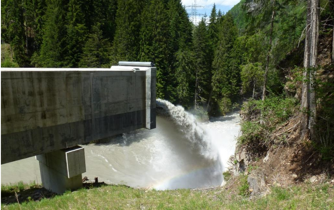
Figure 6: Cantilevering tunnel outlet during operation on May 23 rd 2014 (courtesy of C. Auel)
