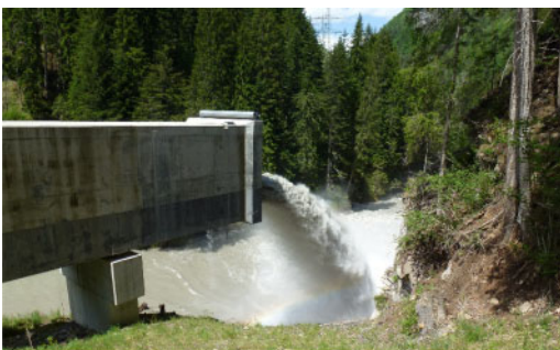
Figure 1. Outlet of the Solis SBT (courtesy of C Auel).
