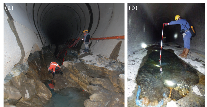
Fig. 3 Abrasion patterns at a) Palagnedra SBT, Switzerland and b) Asahi, Japan (courtesy of C. Auel).
