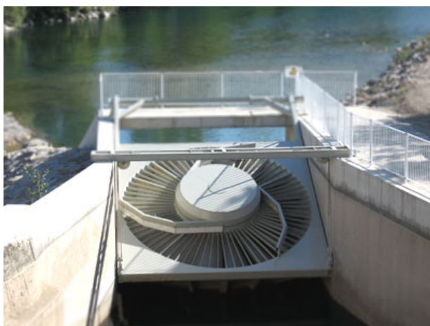
Fig. 2: VLH-Turbine in operation position [17]
