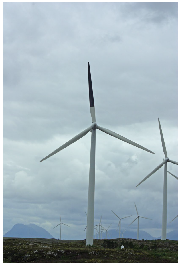
Fig. 1: Wind turbine in the Smøla wind-power plant with painted rotor blade (c) Roel May [1]
