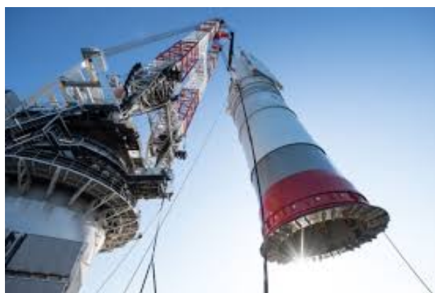
Fig. 4: IHC noise mitigation system, © Ørsted.
