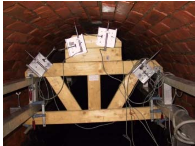
Figure 10. Left: Sectional view of the masonry main sewer with oval shape 1310/1700 mm in Bremen, Above: Measurement base unaffected by the load using 6 linear variable differential transformers (LVDT)
